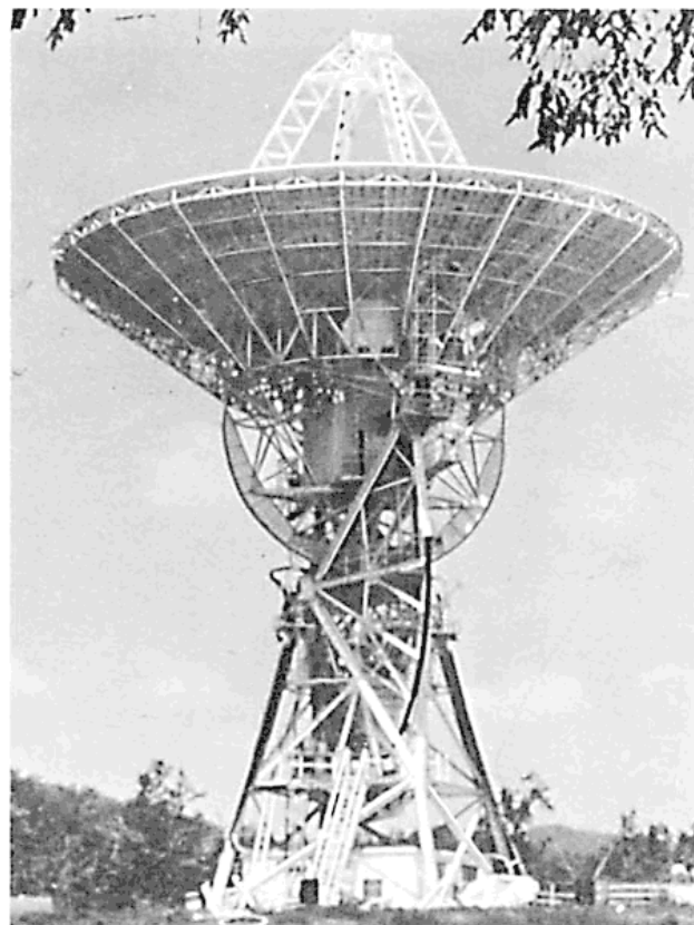
Figure 7—Eighty-five-foot antenna, similar to Apollo antenna.
