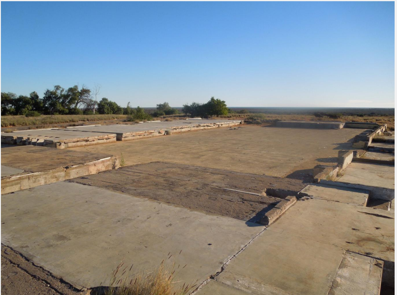
Below: A longer view showing the concrete foundations of the T&C building.
