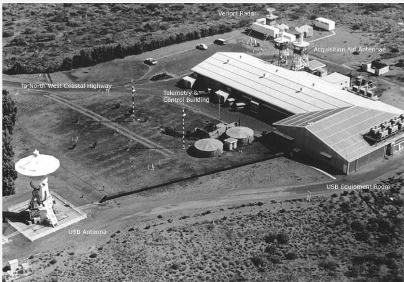
Below: An annotated aerial view of the Telemetry and Control building and surrounding installations.
