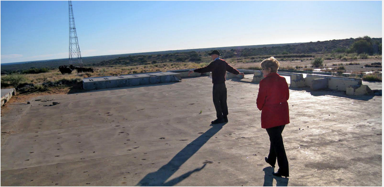
Above: David Johns and Kathy Franin inspect the foundations of the T&C building. The Broadcast Australia tower is visible to the upper left.
