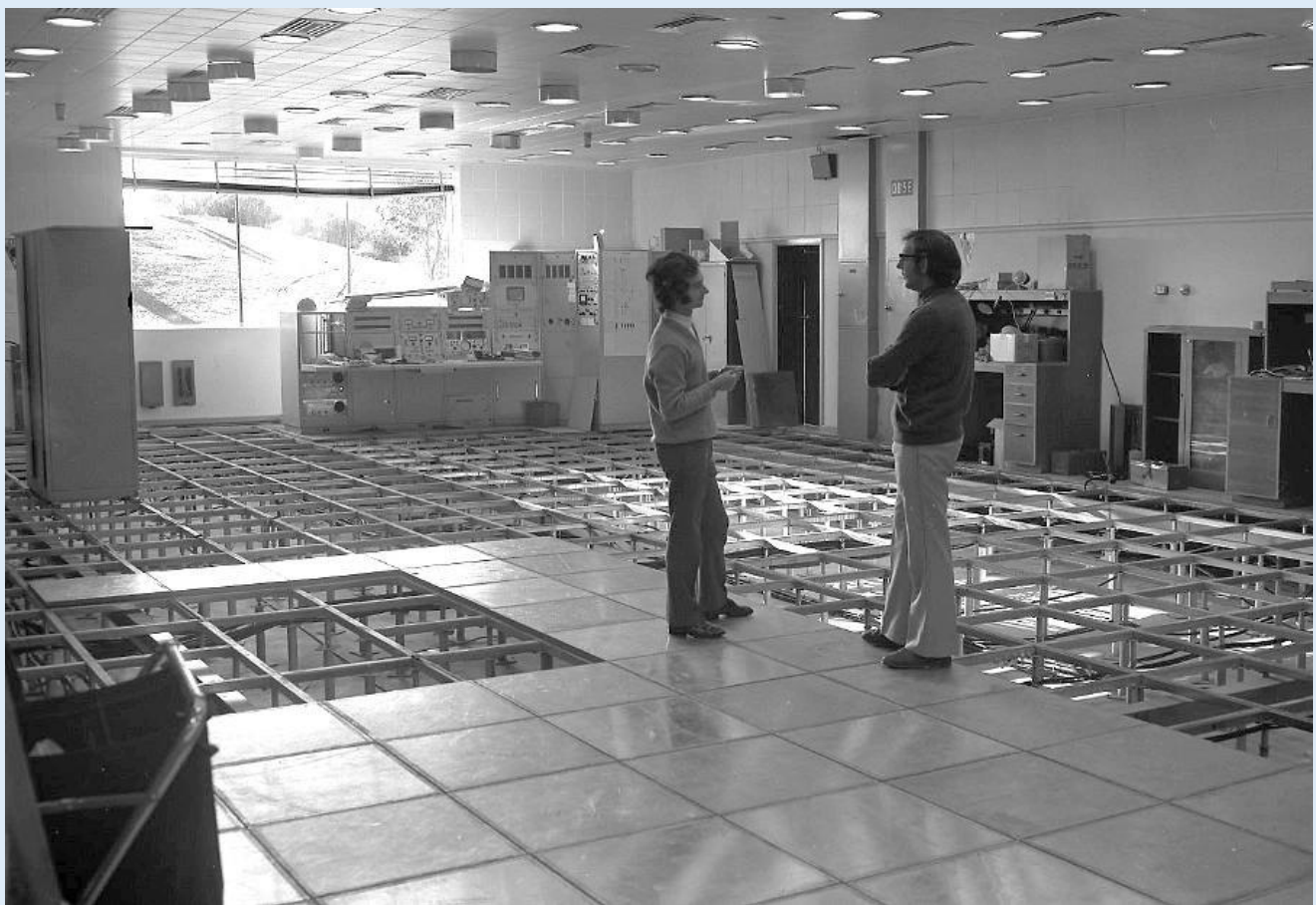
Above: Stirling Finlay (USB) and Charlie Collins (Comms), standing on a completed section of the underfloor cable and air conditioning plenum in the USB area.
