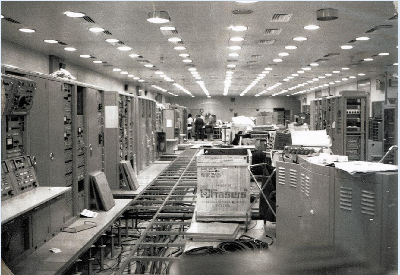
Above: The DSN reconfiguration underway in this photo taken on 134 September 1974.
