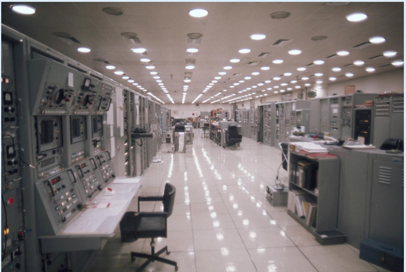
Below: The same view as above after all the new systems were in place.
