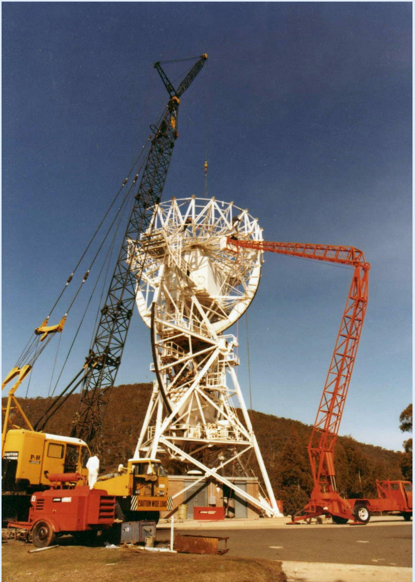
The antenna structure stripped down to the core structure. Photo: Paul Hutchinson Each part of antenna DSS-44 was numbered and colour-coded to allow for parts to be shipped to the Tidbinbilla station for re-assembly, reconfiguration, and a new life as DSS-46.
