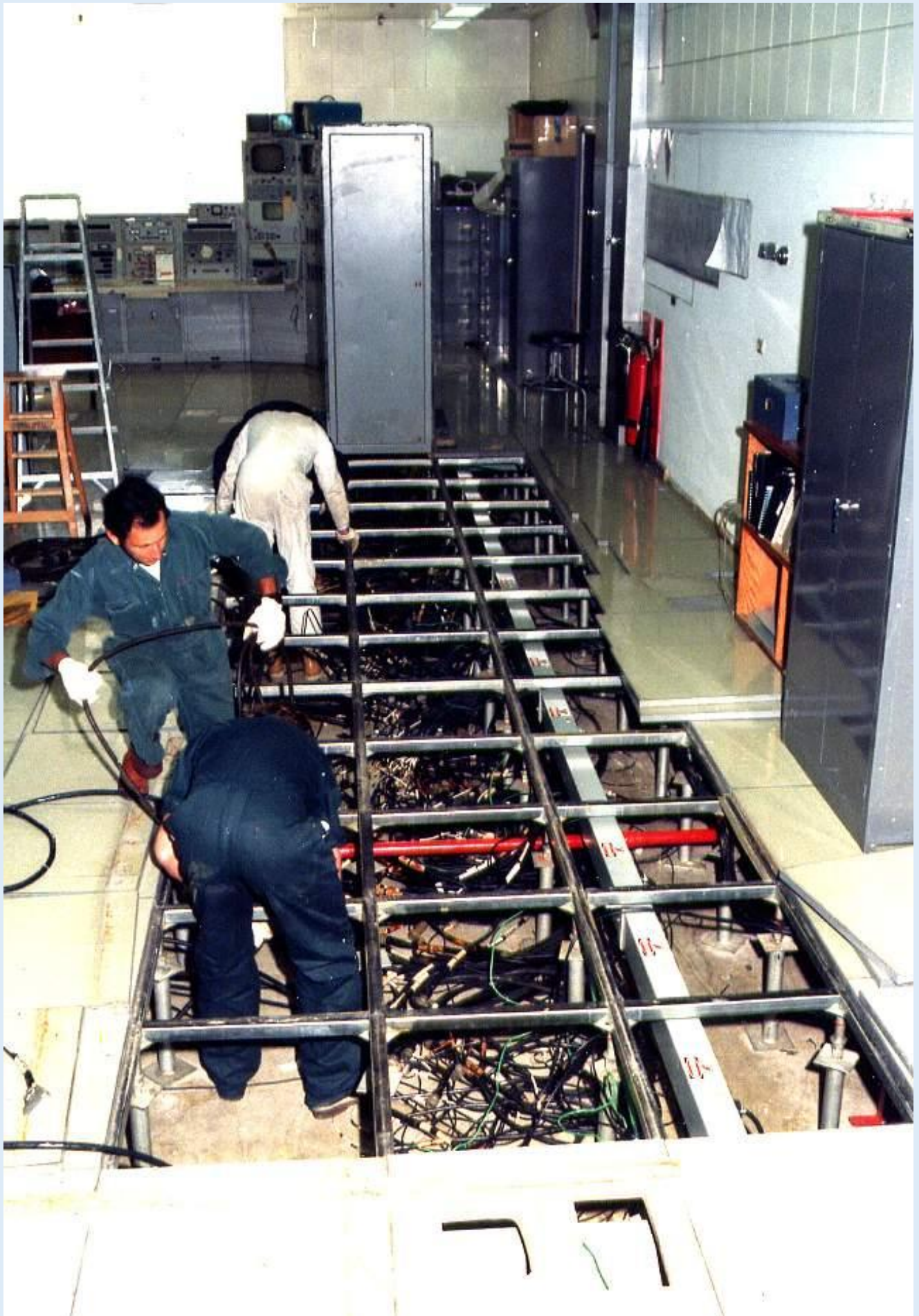
Staff removing cables under the plenum - Alex Sommeriva facing camera. The Receivers have been removed. The Servo console is visible in the background.
