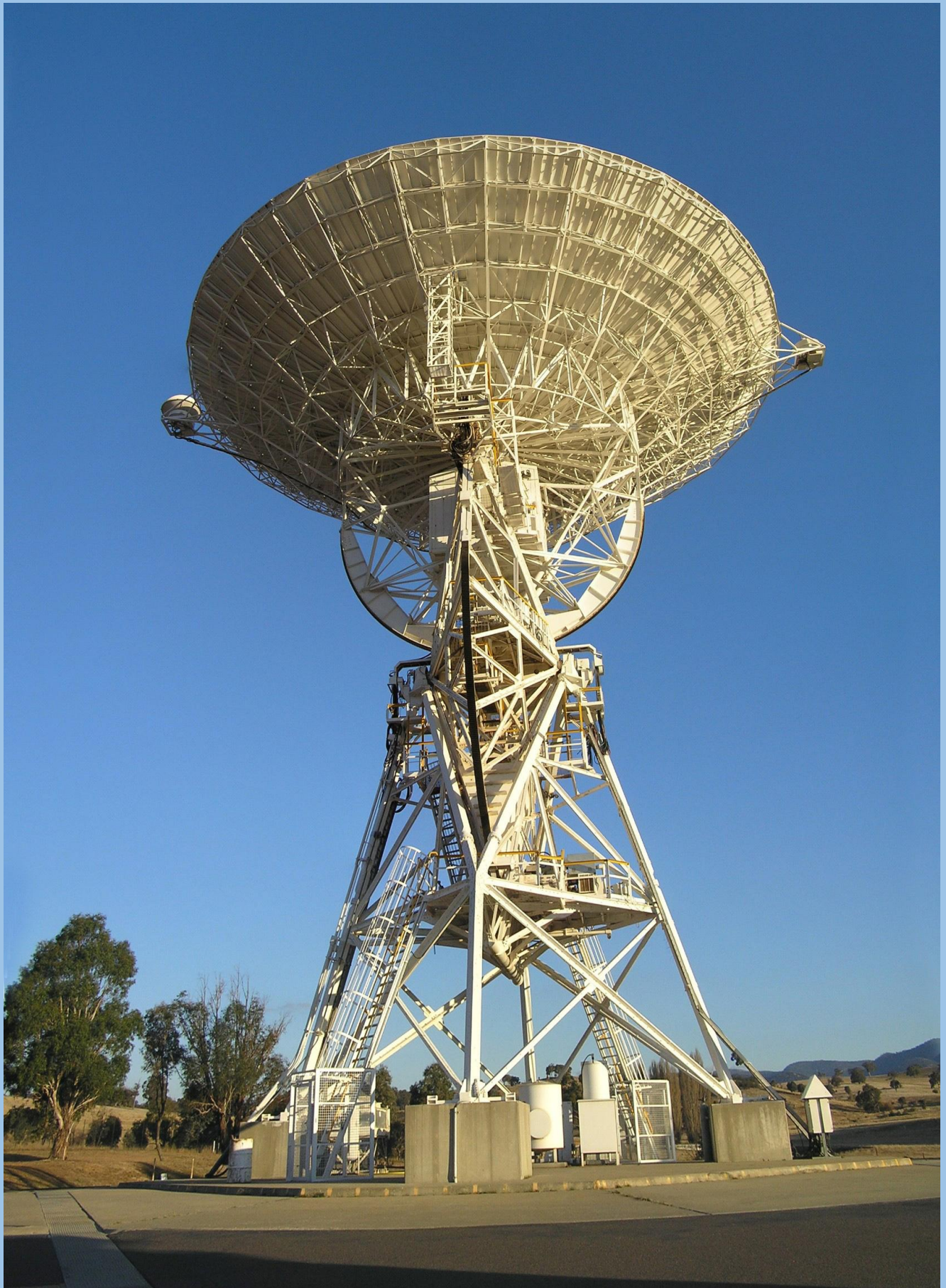
The Honeysuckle Creek antenna in its current incarnation as Deep Space Station 46 (DSS-46), now stands 'retired' at the Canberra Deep Space Communication Complex at Tidbinbilla. After being moved from Honeysuckle in 1981 as DSS-44, it was reconfigured for ongoing Deep Space Network operations at Tidbinbilla from 1983 to 2010. Photo: Colin Mackellar.
