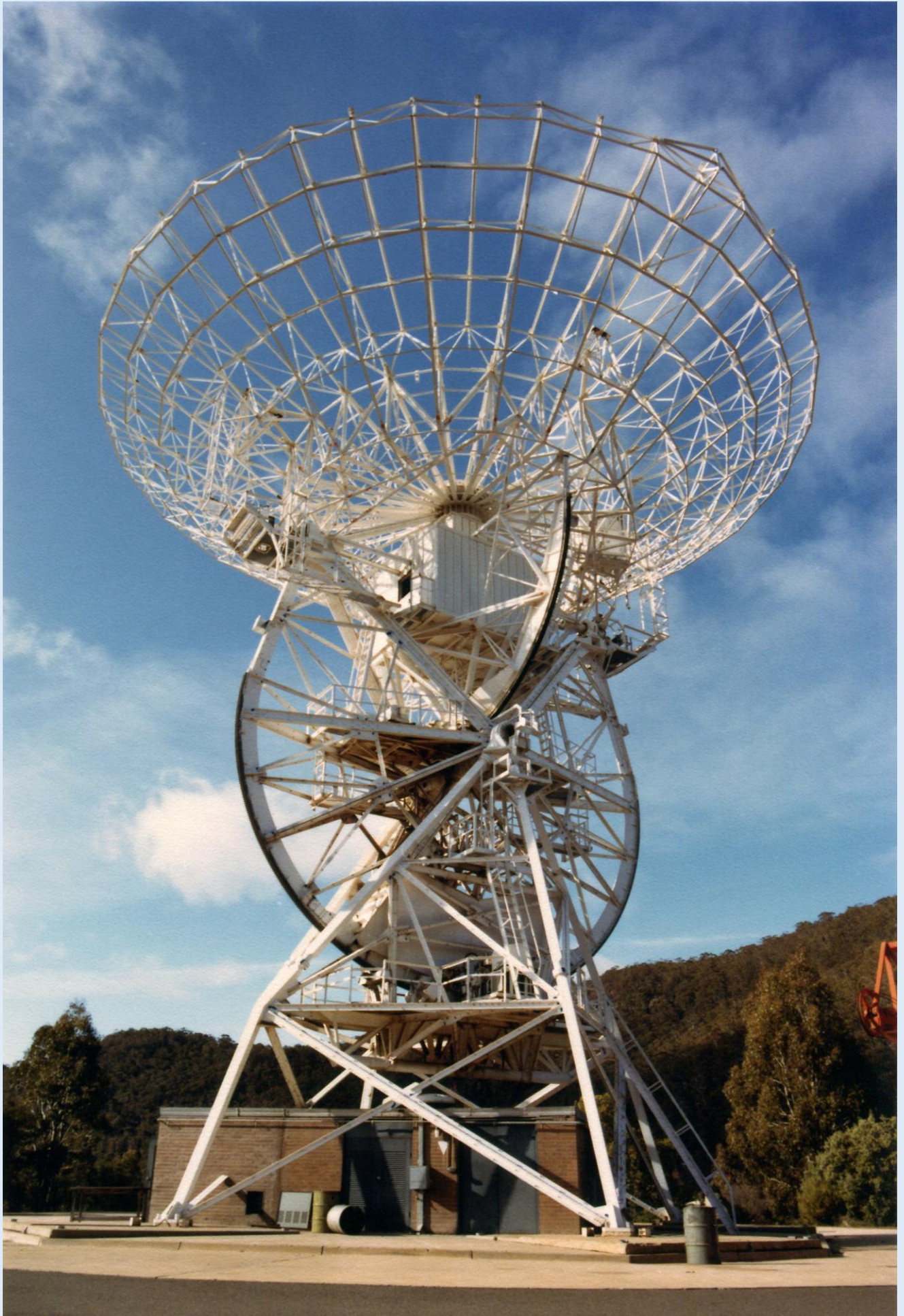
The Honeysuckle antenna is stripped of its reflector panels, as deconstruction begins. Scan: Glen Nagle
