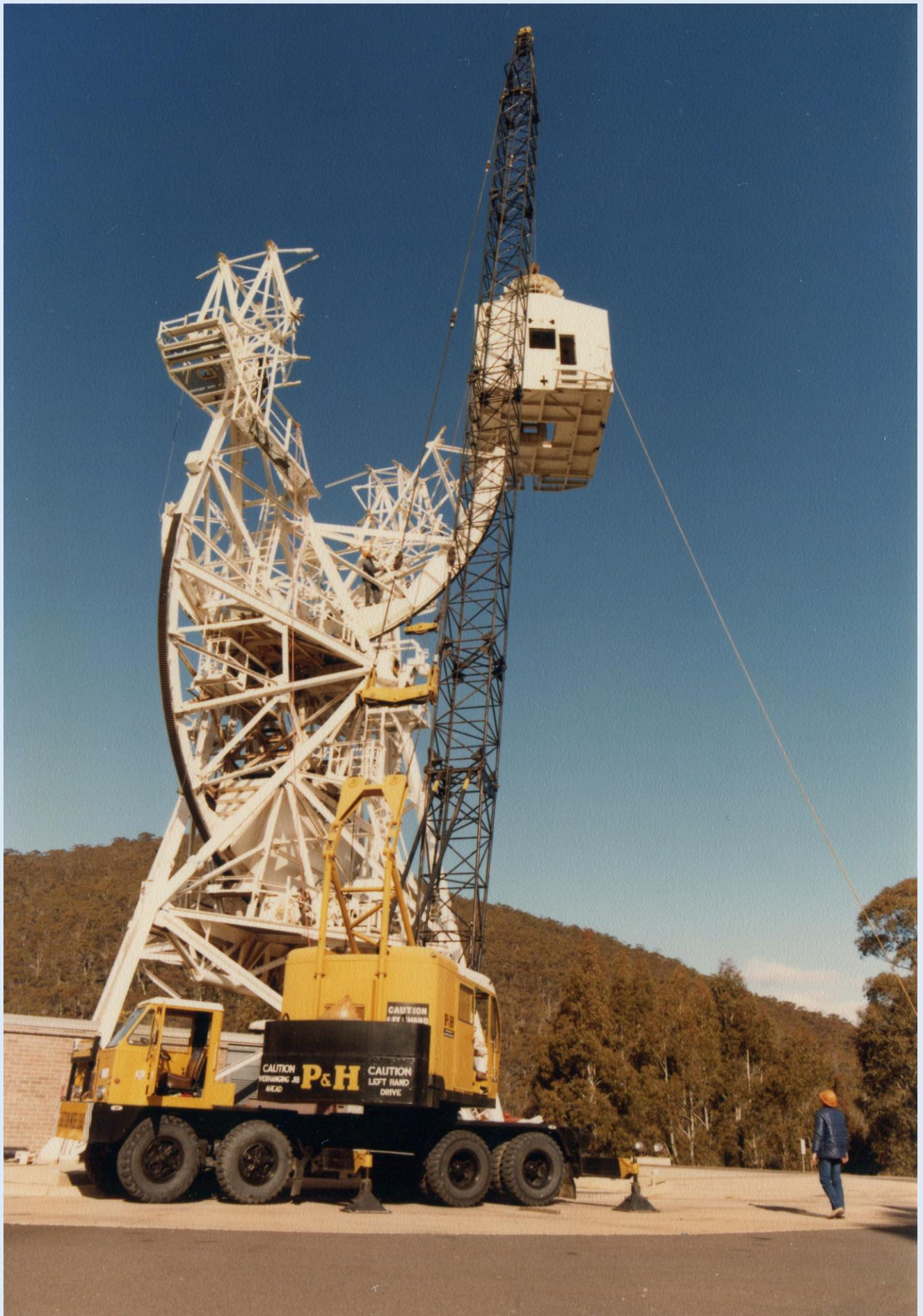
The electronics housing cabin is removed from the antenna. Photo: Paul Hutchinson
