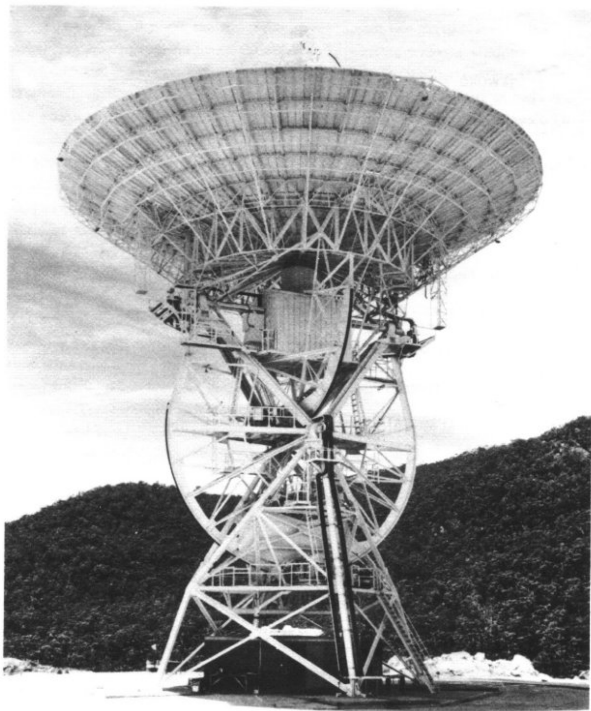
THE 85FT. ANTENNA AT HONEYSUCKLE CREEK
