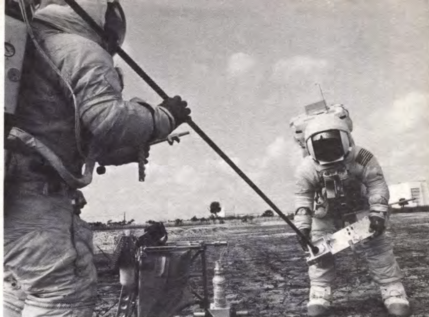
EXPERIMENT PRACTICE. Fred Haise (left) and James Lovell adjust a portion of the heat flow experiment which contains a drill to penetrate 10 feet into the Moon's surface.
