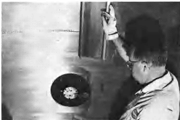
Gibbs is shown inside the chamber during the final boring to size. Note the series of \frac{1}{2} -inch holes.
