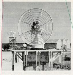
Solid spun-metal type parabolic Verlort antennas are being replaced by expanded-metal type antennas built by the Canoga Corporation. The new antenna has considerable less wind drag than the solid type, and has negligible lift. This change results in a reduction of inertia, which in turn results in less wear and strain on the pedestal. Tracking errors resulting from wind gusts will also be reduced.
