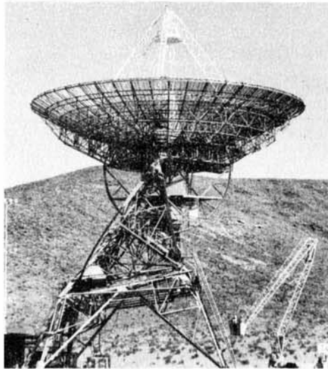
This 85-foot polar mount antenna will provide backup support to the MSFN Apollo USB station at Goldstone, Cal. It is one of three antennas in the Deep Space Network that will serve as dynamic standby stations to the MSFN deep space facilities. The others are at Canberra, Australia and Madrid, Spain.
