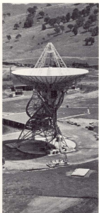
The radio signal, greatly reduced in strength because of the distance it travels, is captured by the Earth antenna.
