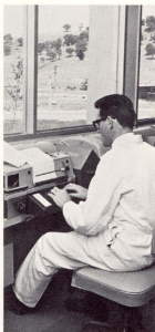
Data gathered at Tidbinbilla are transmitted to the SFOF at JPL by teletype and high-speed digital data circuits.
