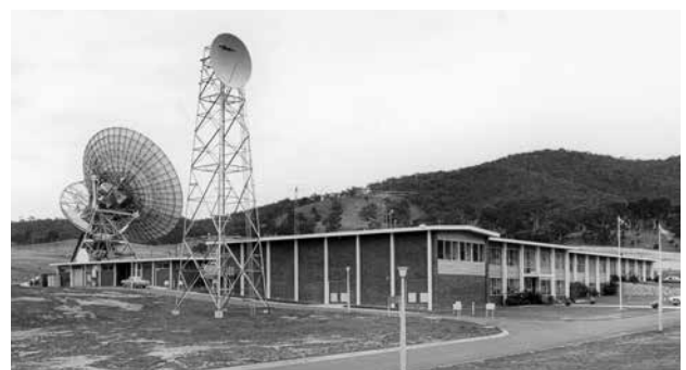
The microwave link tower in its original location adjacent to the new Comms Centre
