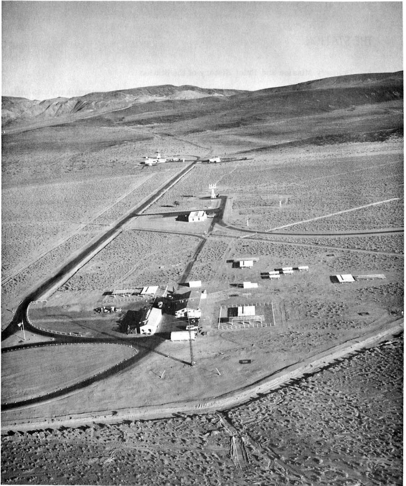
Goldstone Mojave STDN Station
