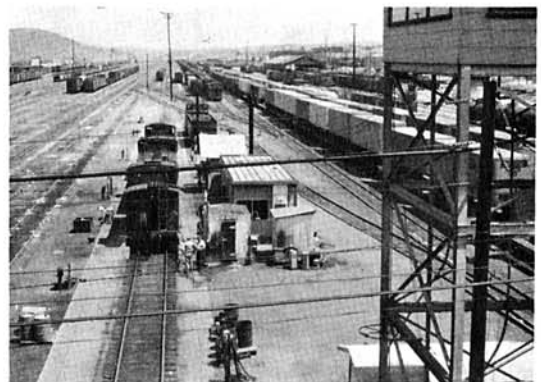
Santa Fe Switching Yard
