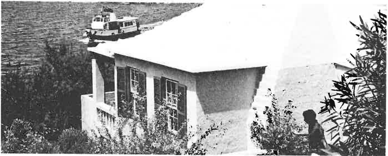
A Gleaming White Roof to Catch Rainwater, in a Typical Bermuda Scene
